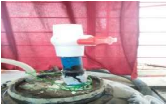
Fig.3 Inlet of digester
